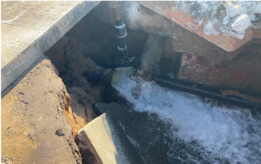
FIGURE 1 – COLLAPSED 12" WATERLINE
